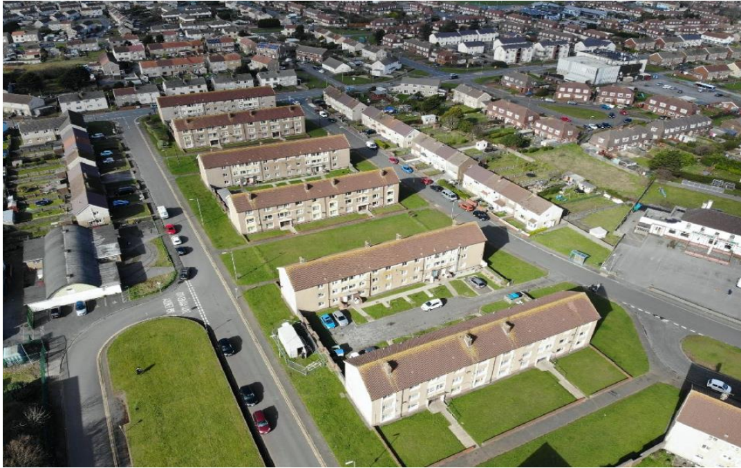
Figure 2: Aerial photo of existing flats
